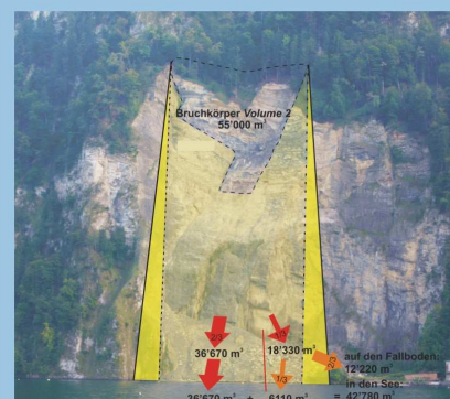
Fig. 7 Actual state of the quarry base.
