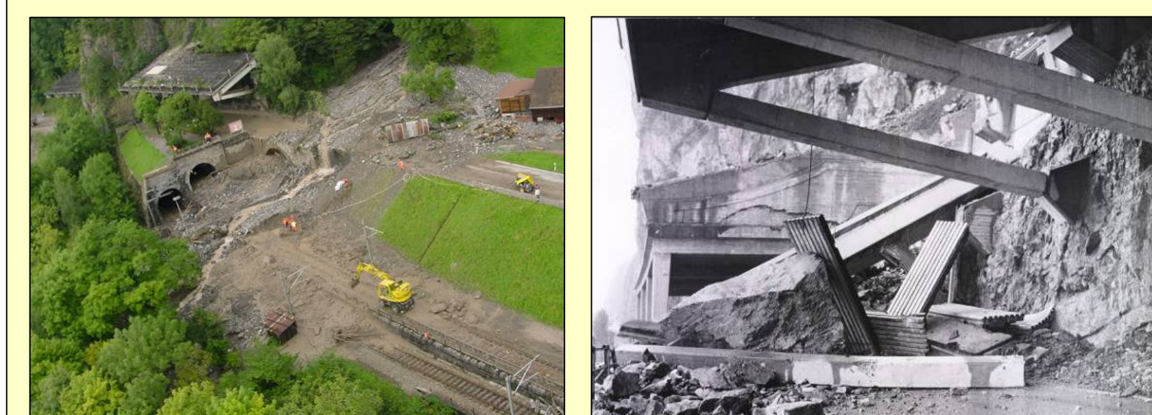
Fig. 3: Left: 2005, Dornibach, debris flow covers highway and railroad. Right: 1970, Rockfall gallery destroyed by rockfall event (500-600 m 3 ).
