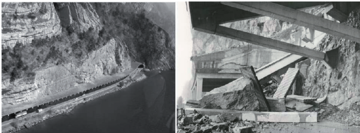
Fig. 1: Part of the Axen national highway with rockfall protection gallery (left). Gallery destroyed by rockfall event (500-600 m 3 ) in 1970 (right).
